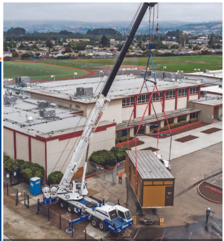
Modular Building Install - John Muir Middle School
